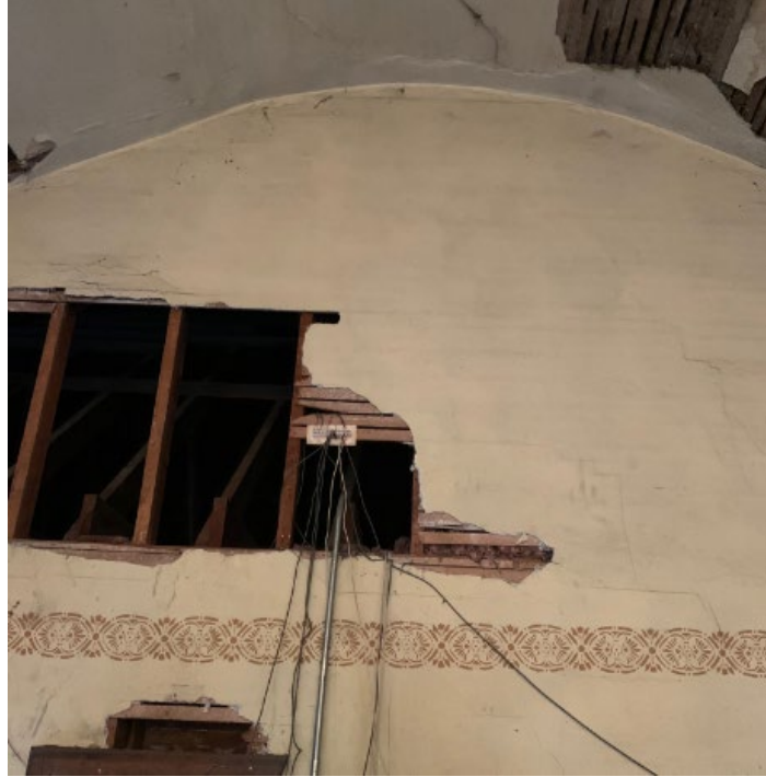
1892 twenty-foot vaulted barrel ceiling from above 1917 false ceiling.
