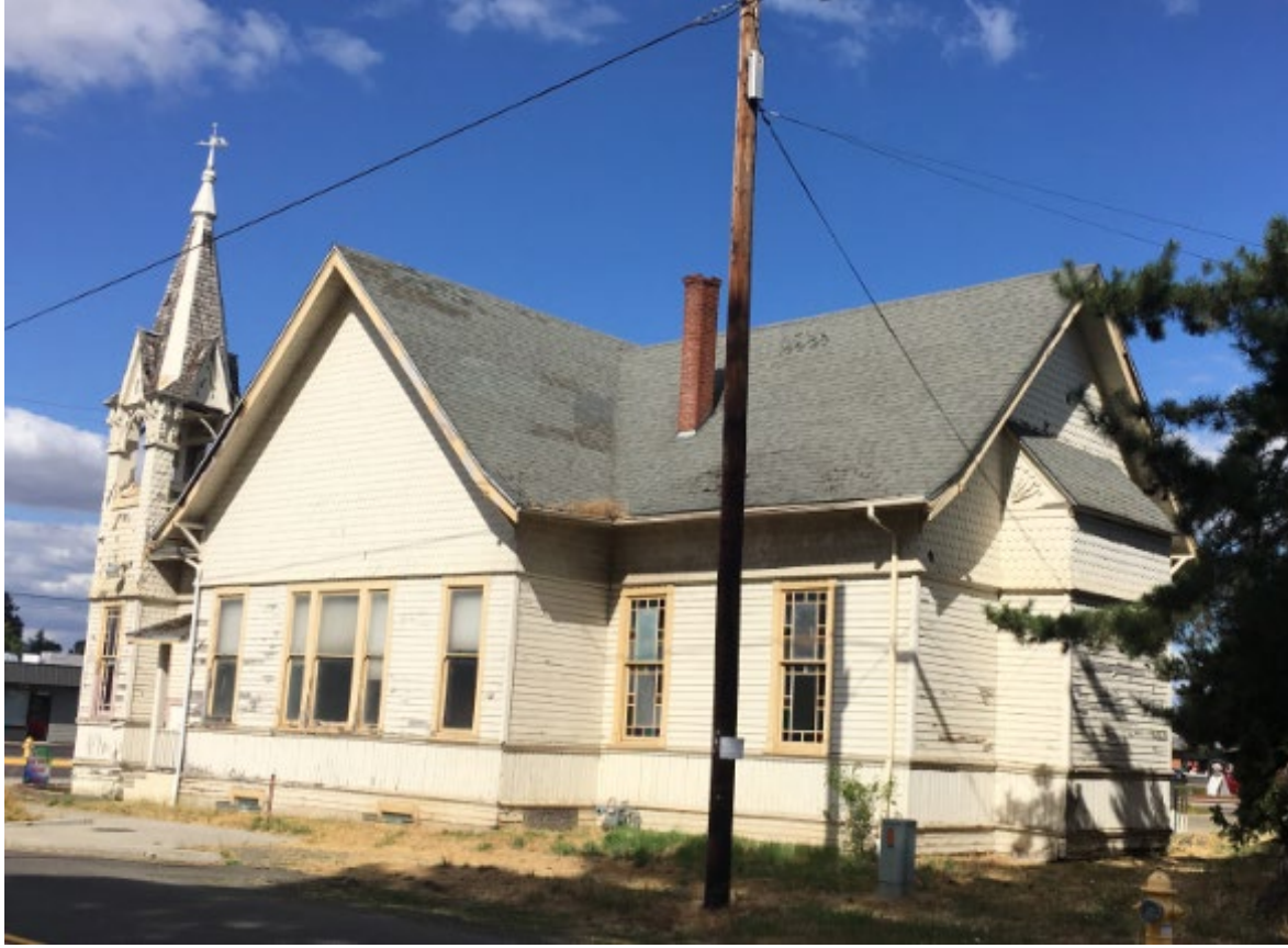
West side church view. Note quarter sunbursts and octagonal imbricated shingles above apse extending at south (rear) of building.
