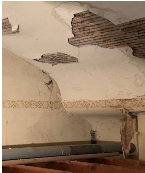
1892 north and south end vaulted ceilings from false ceiling added in 1917.
