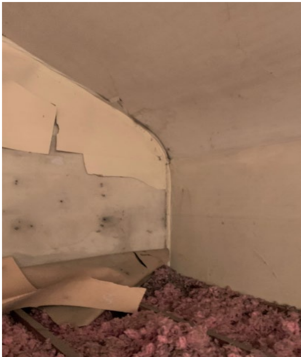
1892 north and south end vaulted ceilings from false ceiling added in 1917.
