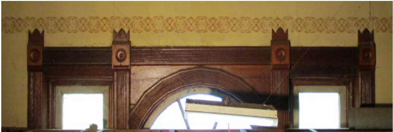
Unstained interior fluted window casing for ganged window unit, on north front of church. Top half of wheel window with arched fluted casing visible. Decorative crowns top the rosette style corner blocks.
