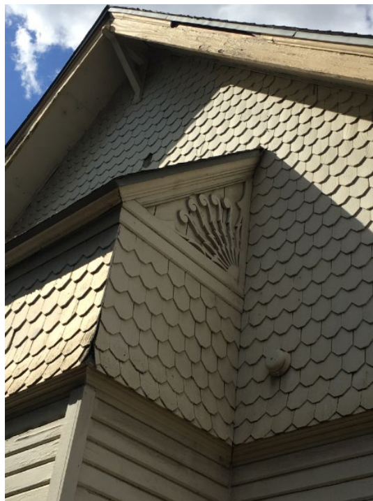
West side church view. Note quarter sunbursts and octagonal imbricated shingles above apse extending at south (rear) of building.
