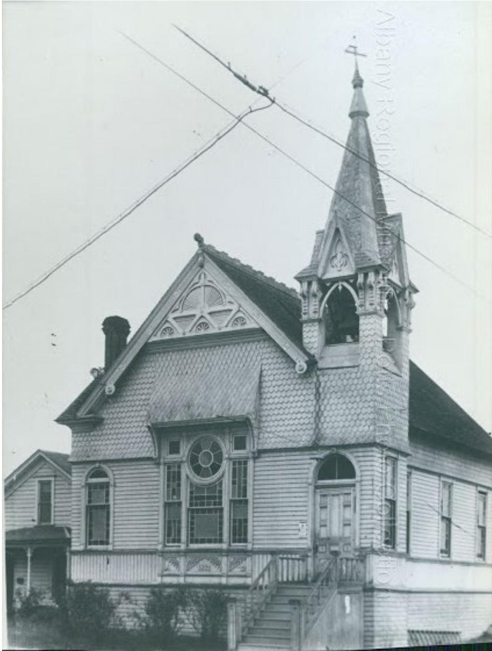
1892 church with brick foundation which raised church 5'-6' above street level. Front gable peak has decorative curved finial.
