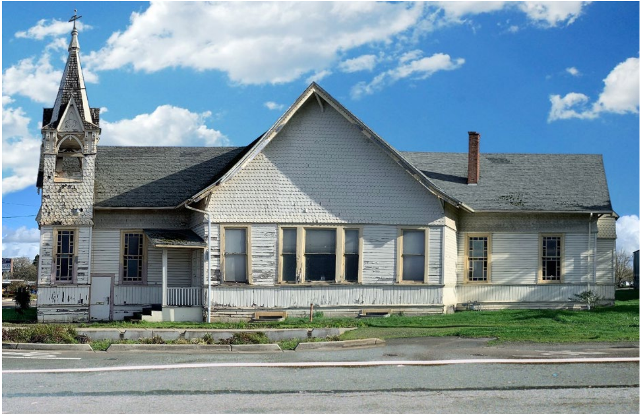
West side of church showing 1892 construction on both ends and cross gable section with new entry added in 1917.
