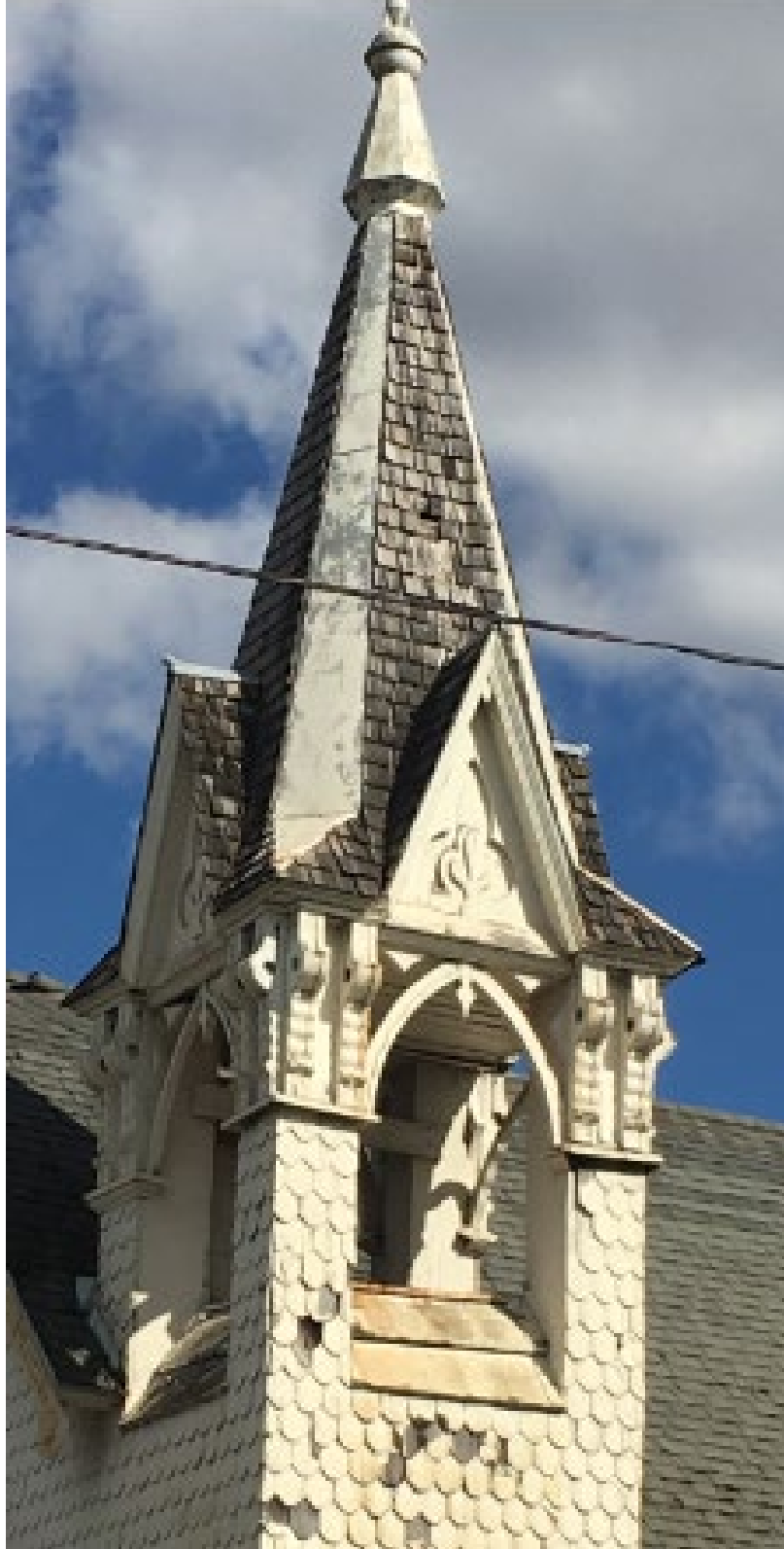
Open side steeple with Eastlake scrollwork at northeast corner of church.
