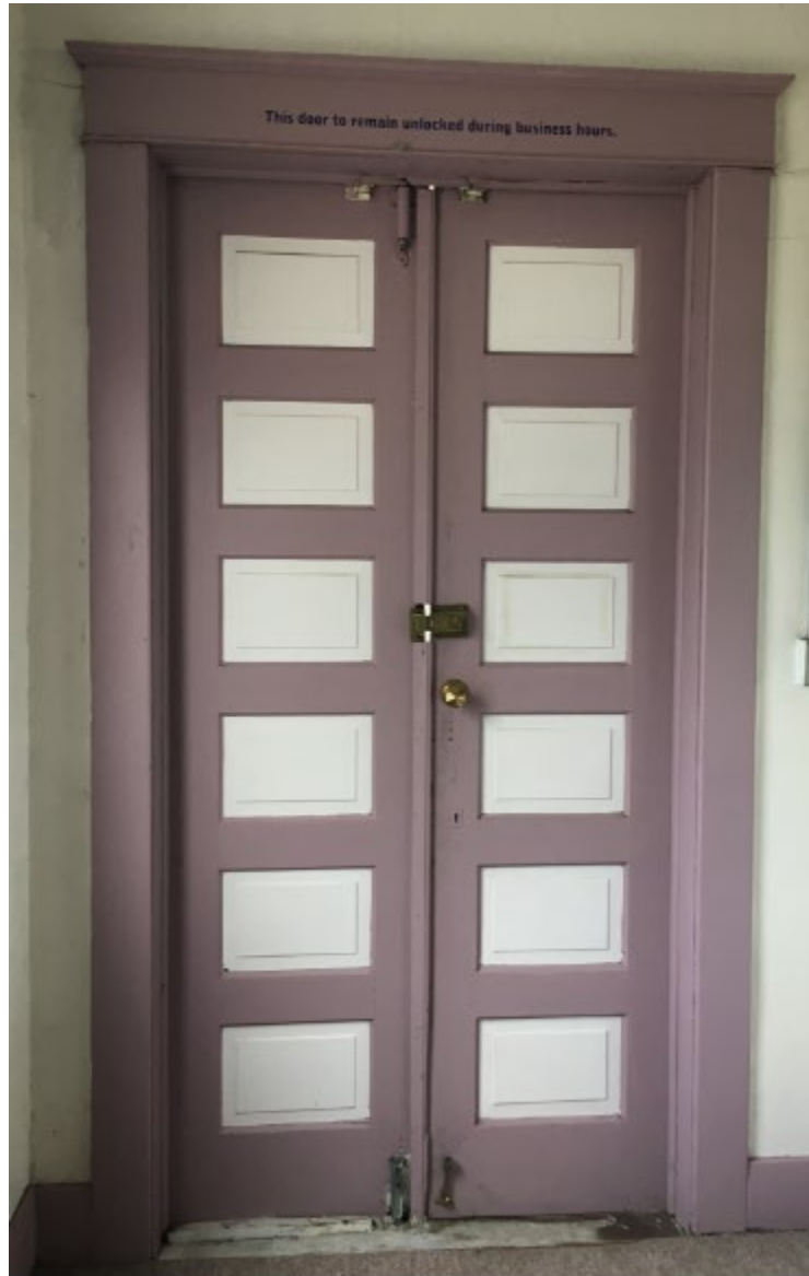
1917 interior entry doors vestibule to nave
