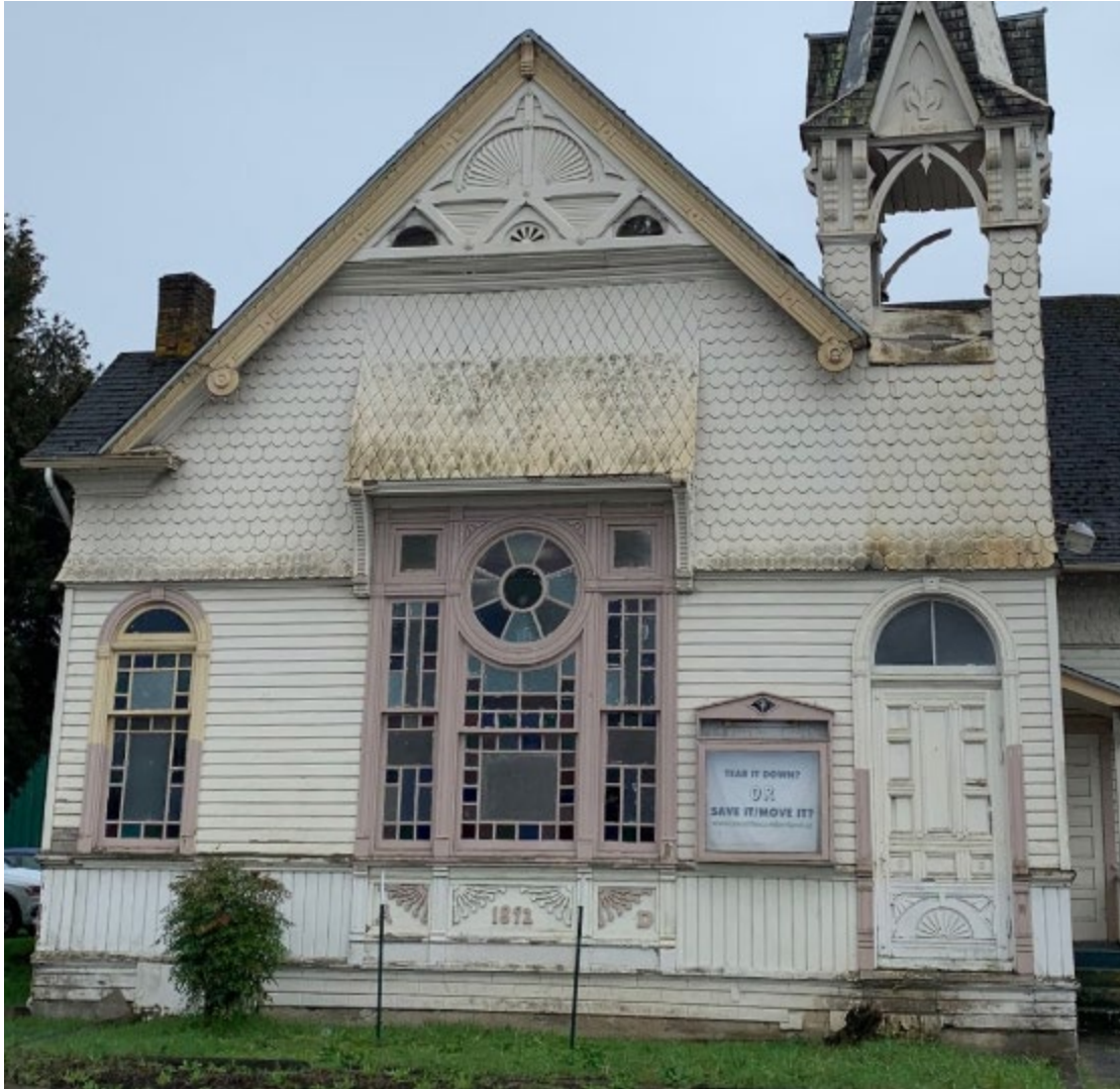
Church front, north side along Santiam Road showing central wheel window and ganged true divided light windows. Original Entry on right side of photograph.
