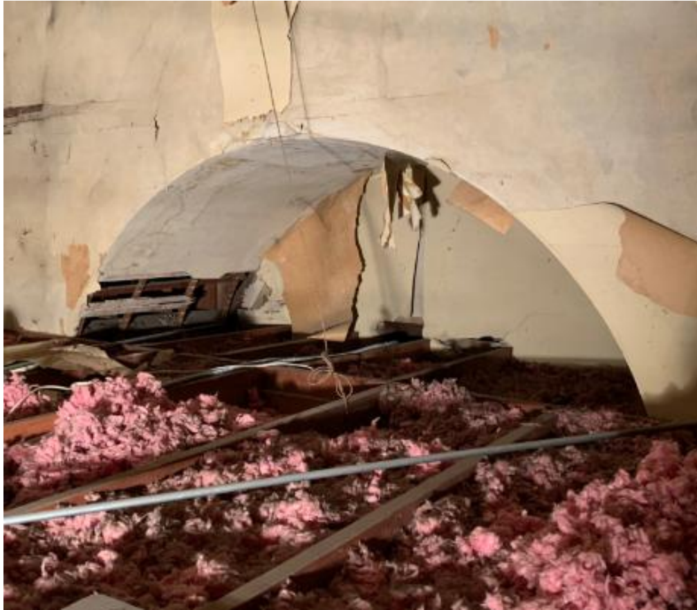
Original semicircle apse ceiling above 1917 false ceiling at south end of church.
