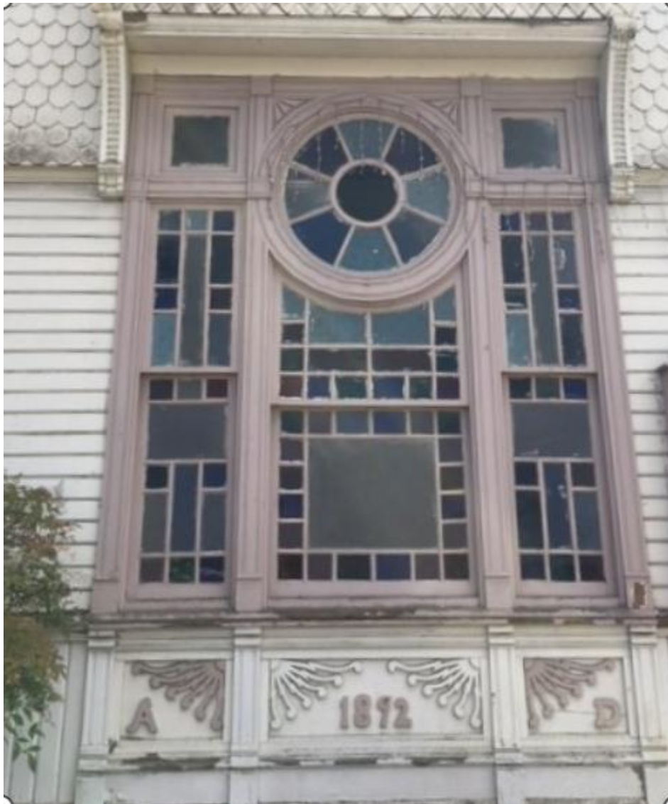
Eastlake ornamentation with sunbursts below window unit showing year of church construction
