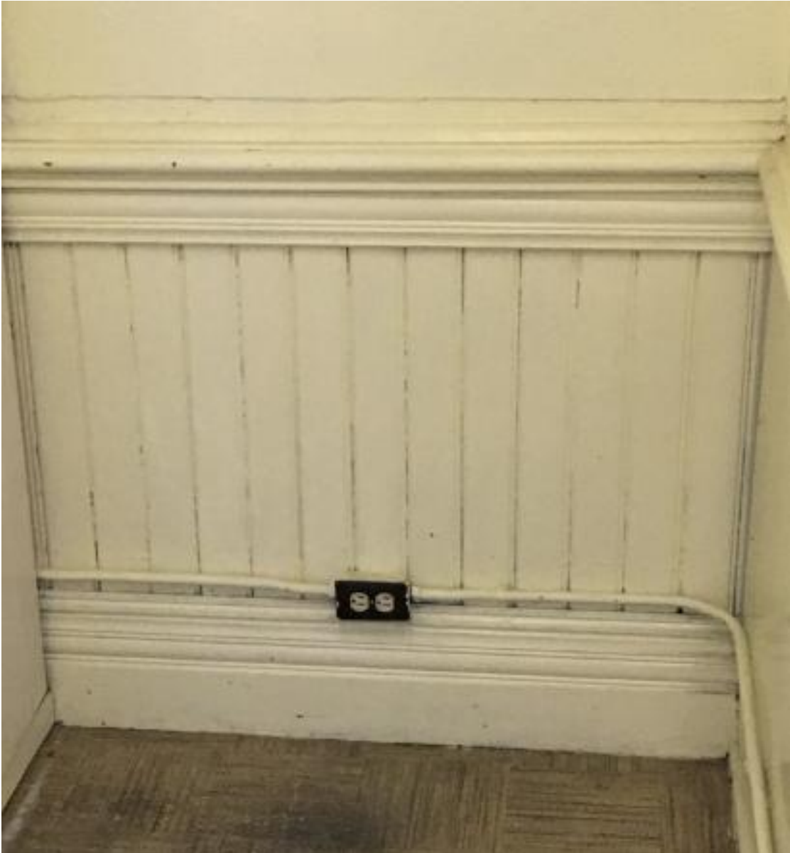
View of wainscoting, chair rail and base (with added electrical outlet)
