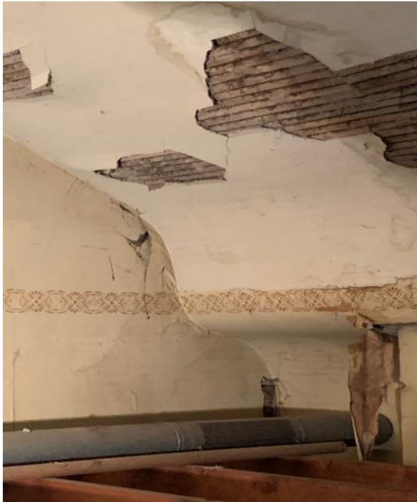
1892 north and south end vaulted ceilings from false ceiling added in 1917.
