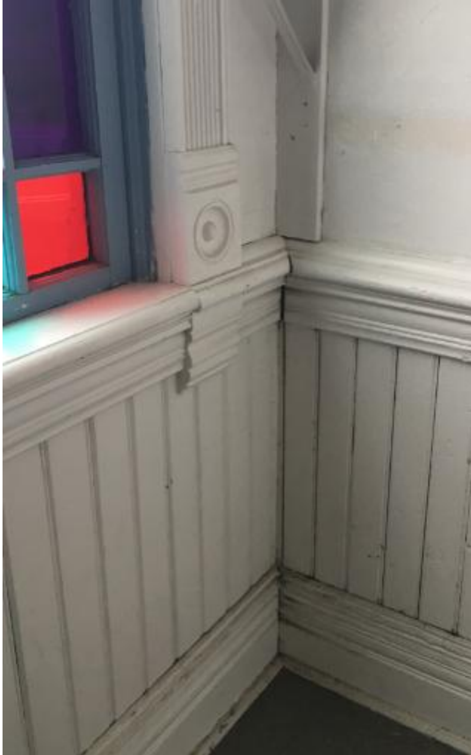
1892 decorative interior mouldings include 9 ½" tall base, 30" tongue and groove wainscoting below 7" chair rail, window apron, rosette plinth blocks and 5 ½" wide fluted casing.
