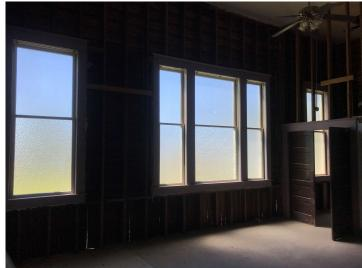
Interior Demolition Removing interior partitions & false ceilings. Removing lath & plaster on exterior walls to expose existing conditions. 350 volunteer hours expended to-date.
